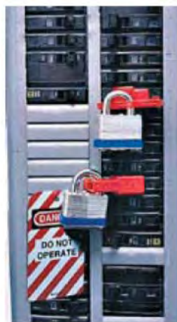
Danger tagged circuit breaker locking off devices
